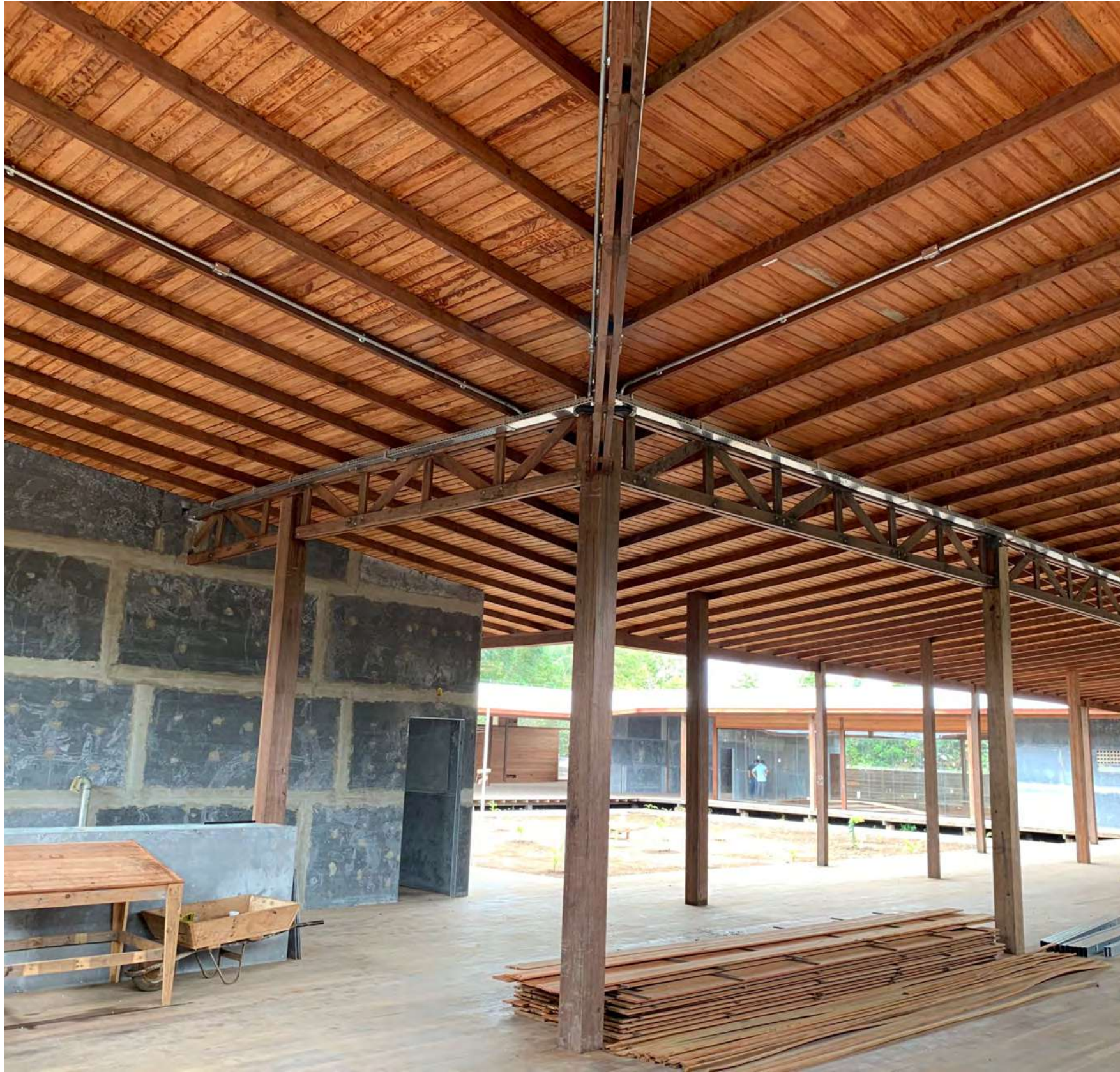
Structure installation: end of the lining installation.
