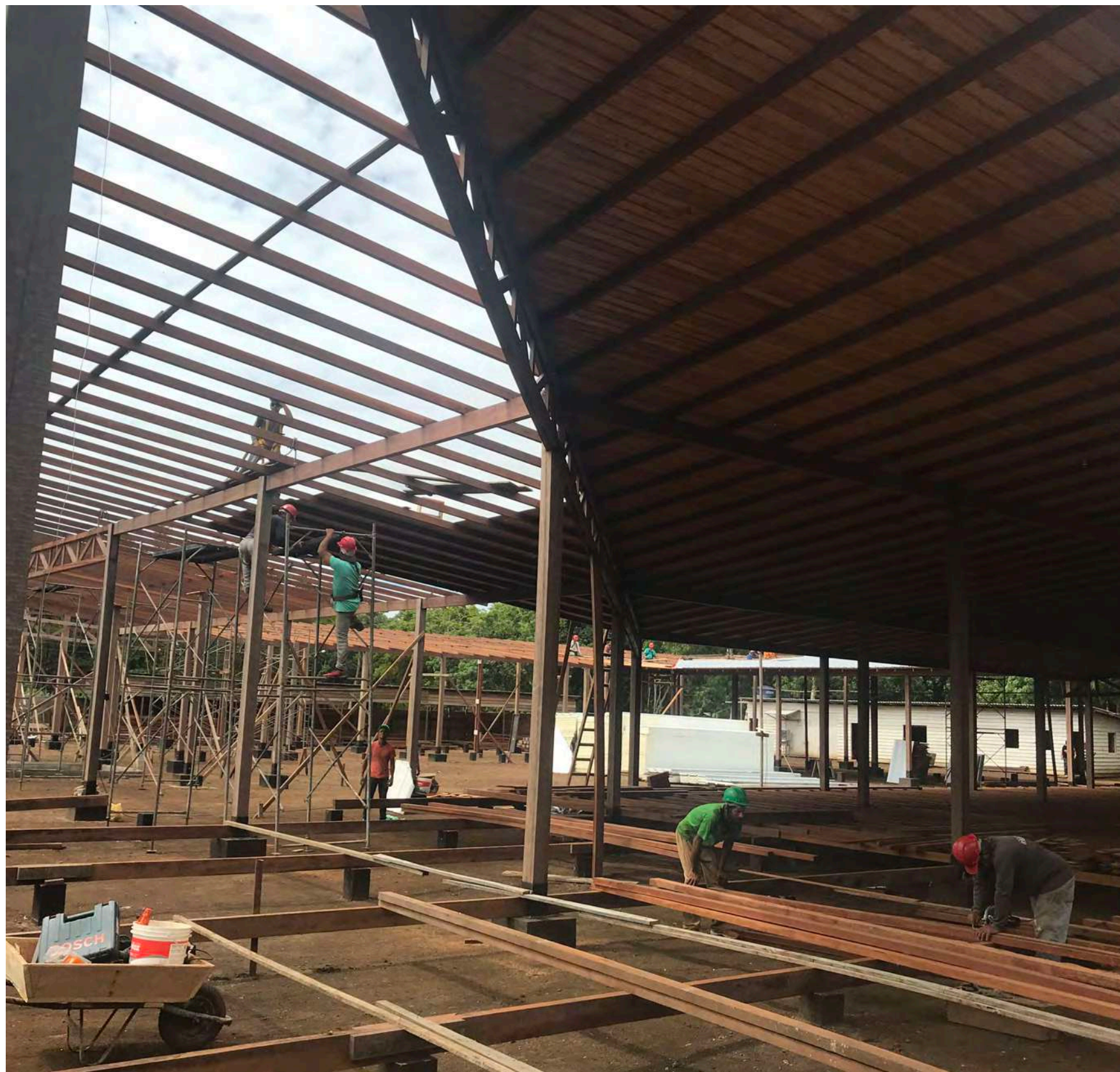
Structure installation: Beginning of the roofing installation
